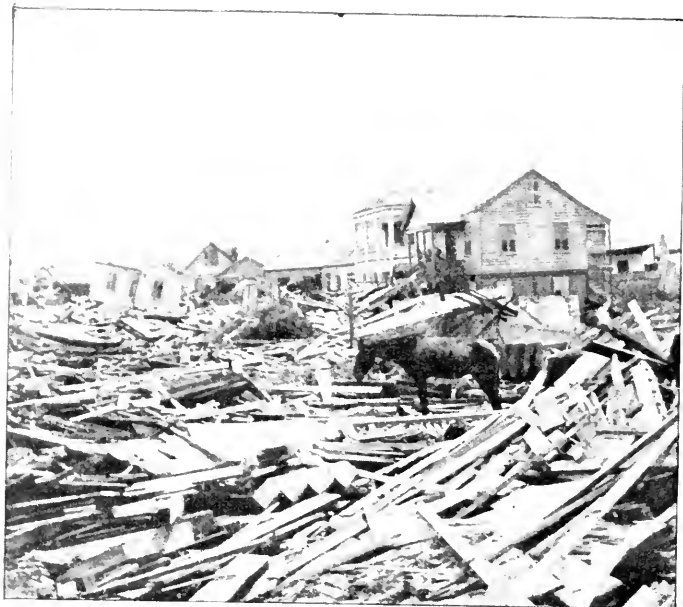
WRECKED RESIDENCES CORNER TWENTY-SEVENTH STREET AND AVENUE M
